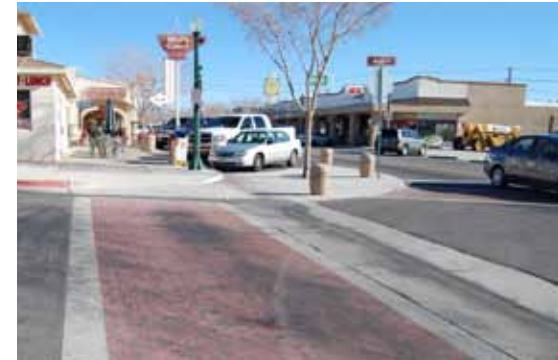
Curb extensions are used as a form of traffic calming. They improve the pedestrian environment by reducing street crossing distances, improving the visibility of pedestrians at street corners, and providing an on-street parking area, which creates a buffer between cars and pedestrians. This curb extension also narrows the automobile travel lane. This helps to reduce automobile speeds, leading to a safer crossing environment for pedestrians.
