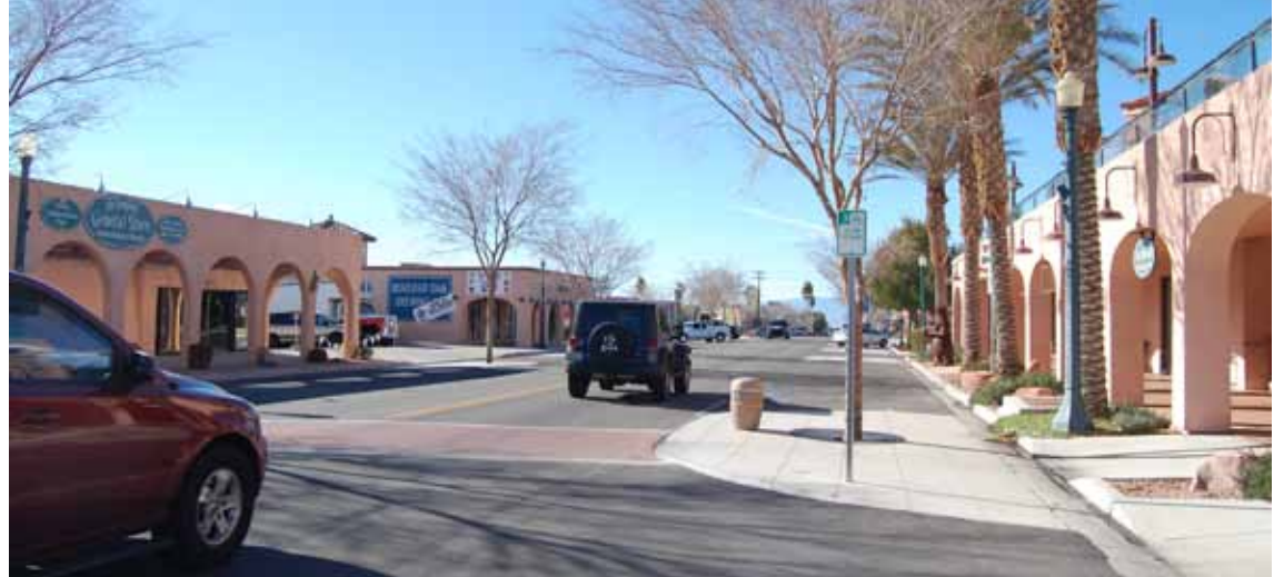
A road diet refers to a reduction in the number of lanes and/or a reduction in lane width in order to achieve improvements to road conditions for pedestrians, bicyclists, or transit riders.
