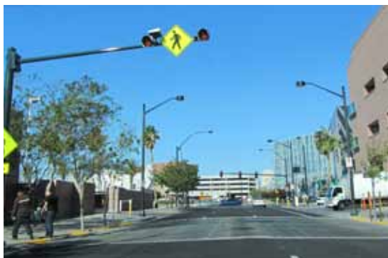
Midblock crossings provide locations for pedestrians to cross streets where the spacing of intersections is far apart.
