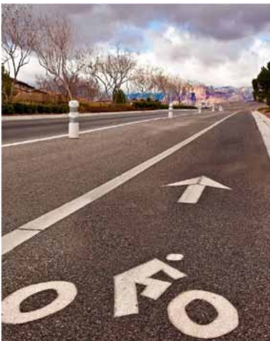
Bicycle lanes are an important component of complete streets, they provide a designated space for bicycles, improve safety, and provide more options for travel.
